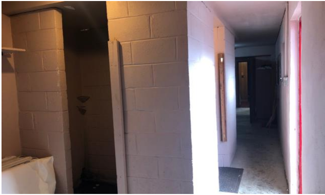
The locker room area was cleaned out before demolition started
