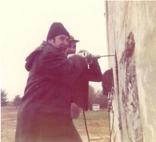
Paul Hoenisch drilling the hole for the kitchen fan
