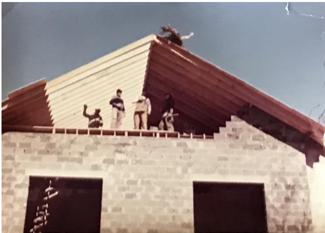
Working on the roof - be careful!
